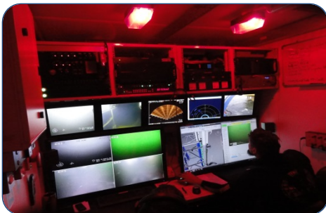
ROV Control Cabin
